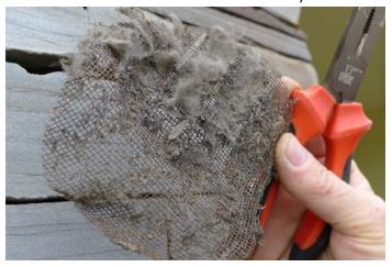
The constant volume fans were running noisily to compensate for the additional pressure loss. The screens were built into the external terminals and could not be accessed for cleaning so the decision was taken to remove them, relying on the easily replaceable prefilter to remove fluff and insects as this filter will be changed regularly.
