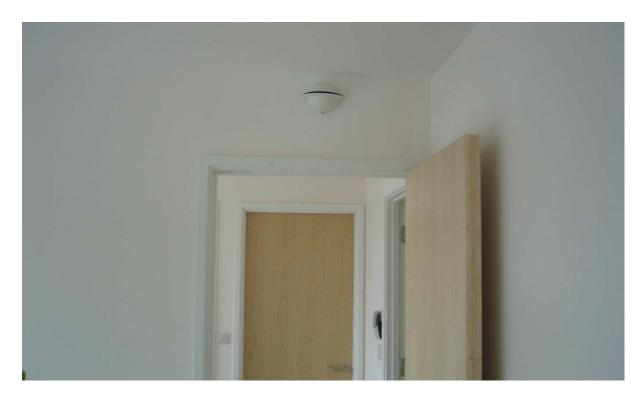
Supply is over doors using a terminal designed to circulate the supply air across the room with the return path at low level under the door.
