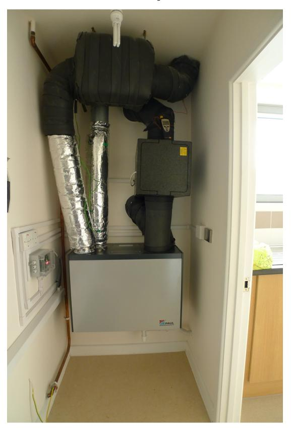
The frost heater is on the right, the silver ducting on the left is silencers on supply and extract, and the heater battery is suspended from the ceiling. The control thermostat for the frost heater is on
