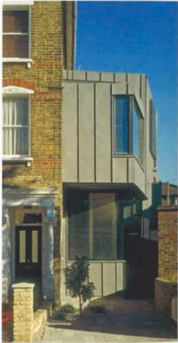
of one another to a thickness of 200 millimetres (8 inches) using a solvent- and formaldehyde-free adhesive, producing incredibly strong panels that can span larger distances than conventional timber. Used for wall, floor and roof slabs, the panels were prefabricated in Austria with window and door openings factory cut, enabling the building to be constructed and fully fitted out in just six months.
