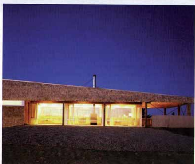
This page Three views of MacKay-Lyons Sweetapple Architects' Hill House: the project consists of a main house and guesthouse/barn separated by a courtyard; ceilings are clad in untreated, rot-proof hemlock which provides a warming contrast to the concrete floors, white walls and large expanses of glass; Douglas fir posts have been used for the colonnaded porches. Opposite Eldridge Smerris Swain's Lane perches on the edge of Highgate Cemetery. The concrete frame acts as an environmental modifier
