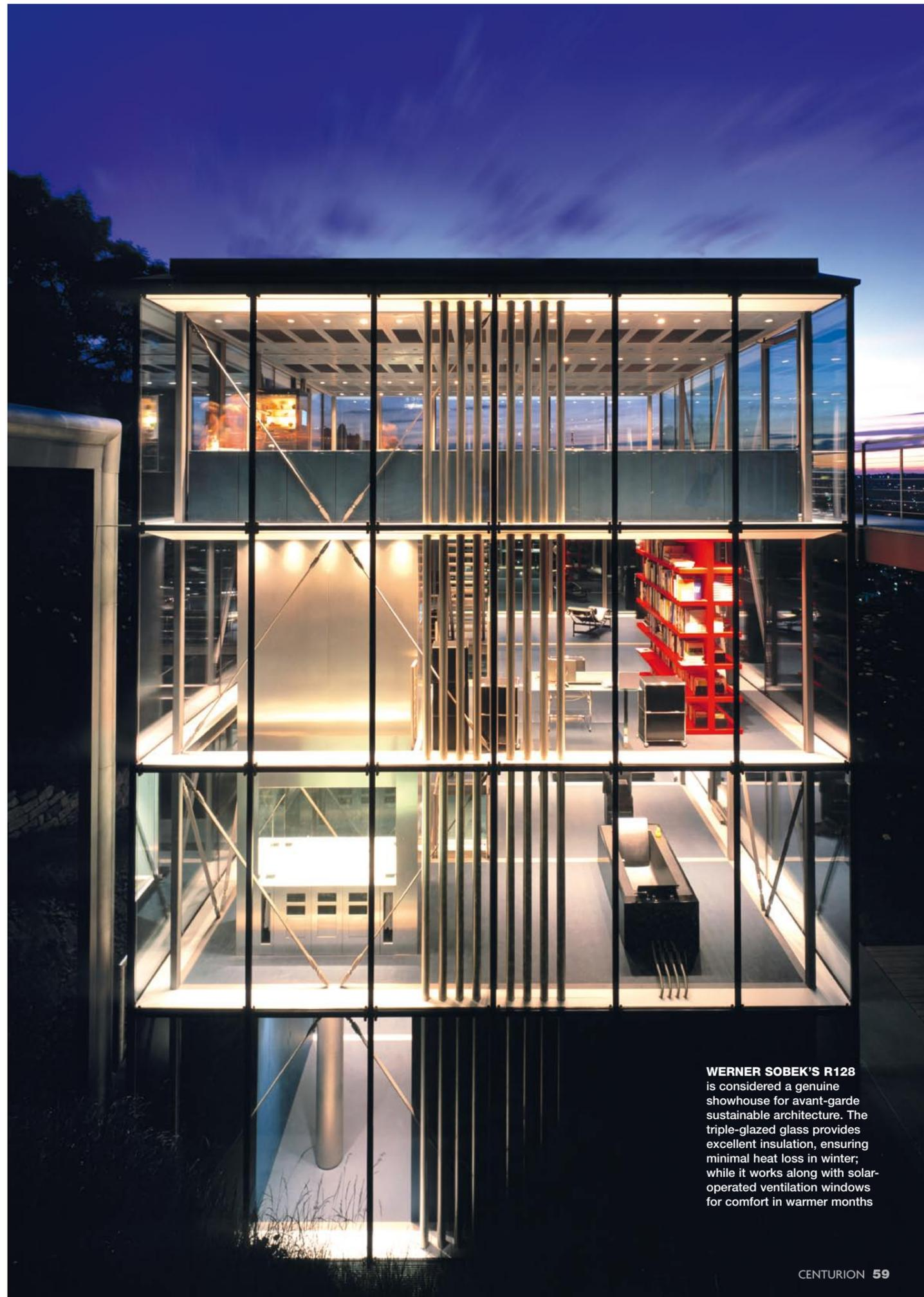
**WERNER SOBEK'S R128** is considered a genuine showhouse for avant-garde sustainable architecture. The triple-glazed glass provides excellent insulation, ensuring minimal heat loss in winter; while it works along with solar-operated ventilation windows for comfort in warmer months
